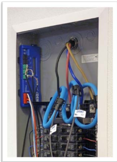
PowerScout 3037 w/R0Coil CTs attached to load
