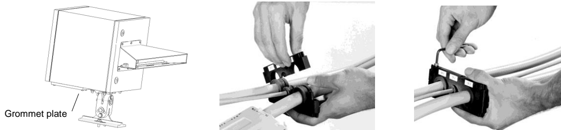
Figure 4-3: Cable Installation
